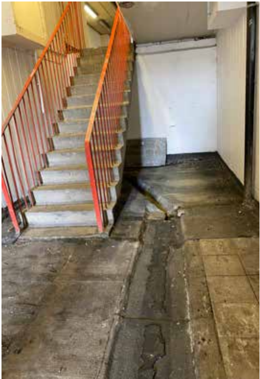
Figure 4.46 Stairwell leading down to car park level under Phase 1 showing defunct drainage channel
