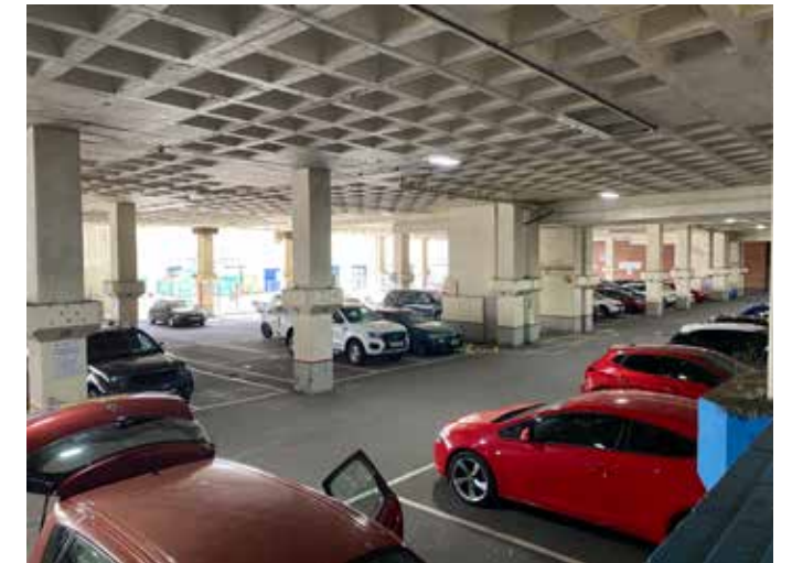
Figure 5.1 Phase 1 Car parking area concrete coffer roof construction
