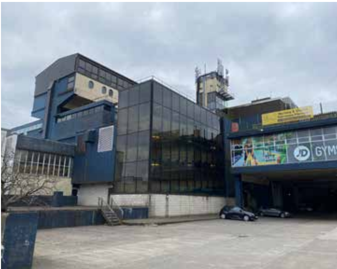
Figure 4.40 Exterior glass cladding over original Phase 1 pedestrian access ramp
