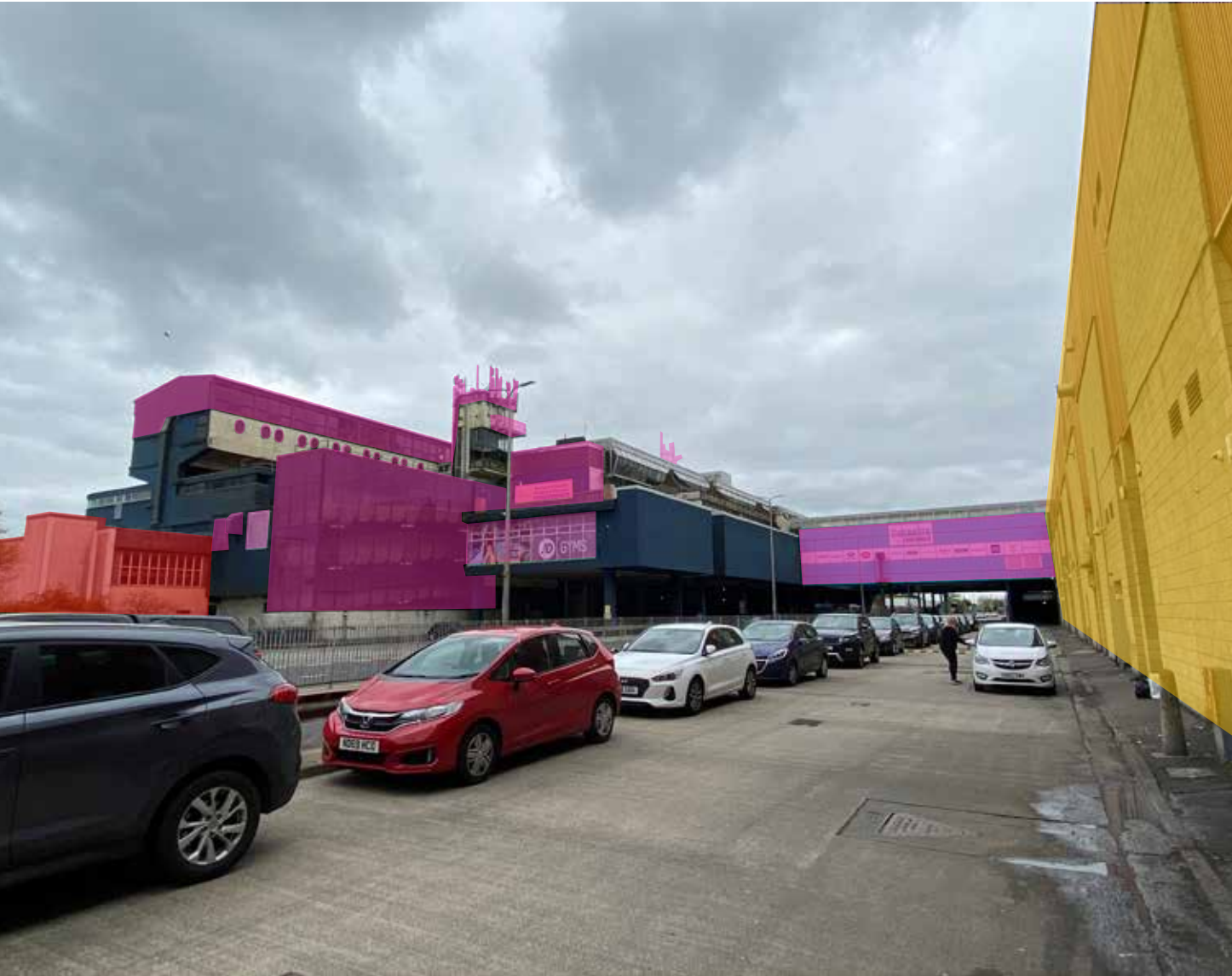
Figure 4.56 Marked up photo of non-original fabric on Phase 1 (east elevation) as well as Phase 3 & 4.
