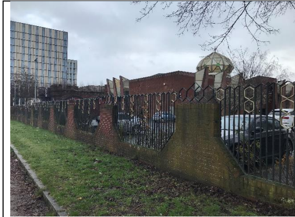
Boundary walls and railings view looking south (16/03/2023) © Historic Environment Scotland
