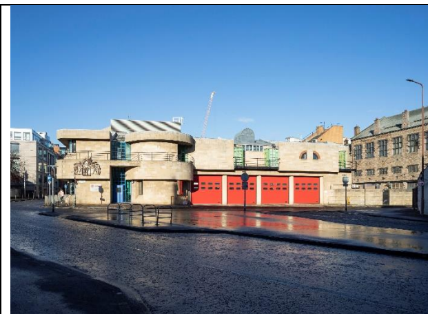
Type: Standard. Title: Tollcross Fire Station, main elevation, looking north. Alternative Text: Tollcross Fire Station, main elevation, looking north, on a clear day with blue sky.
