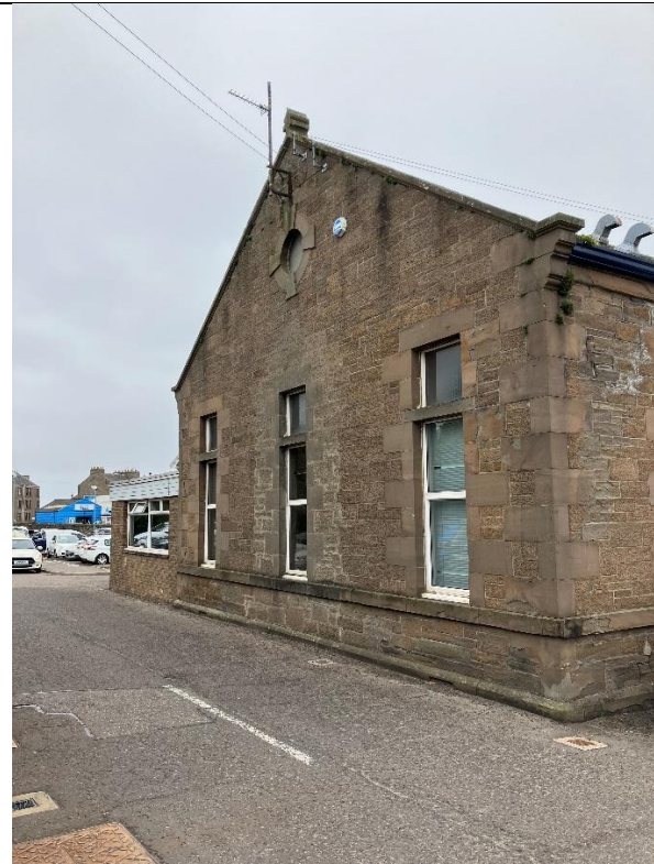
The north gable of an 1889 ward pavilion (31/05/2023) © Historic Environment Scotland
