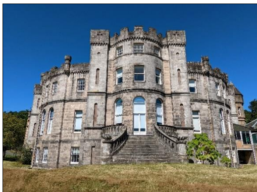
Type: Standard Title: University of Stirling (Airthrey Castle), Airthrey Castle, photographed from the southeast. Alternative Text: University of Stirling (Airthrey Castle), Airthrey Castle, photographed from the southeast, on clear day with blue sky. Date taken: 11/08/2022 Photographer: HES Copyright: © Historic Environment Scotland
